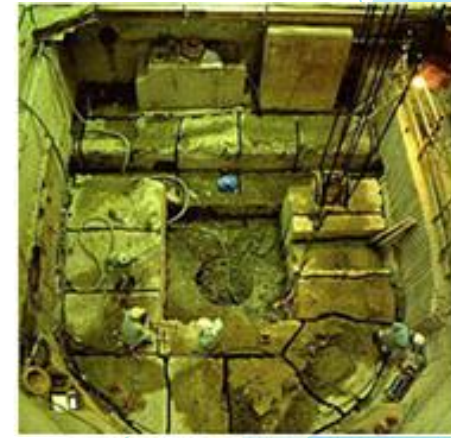
Slots at Basement Concrete
