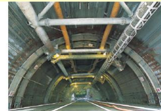
Temporary Shut Off Structure Inside
