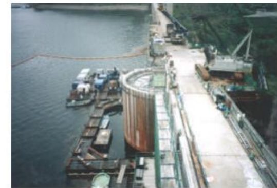
Temporary Shut Off Structure Setting
