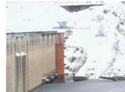
Temporary Shut Off Structure Overview
