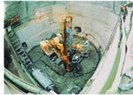
Slot Drilling at Basement Concrete
