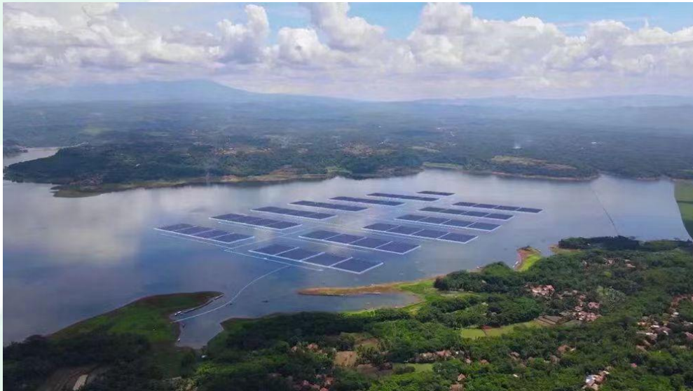
Cirata Reservoir, courtesy Aries Firman 145 MWp ; 200 ha on a dam reservoir of 6,000 ha surface area Cirata HPP : 1 GW ; concrete-faced rockfill dam
